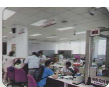
CCTV In Bank
